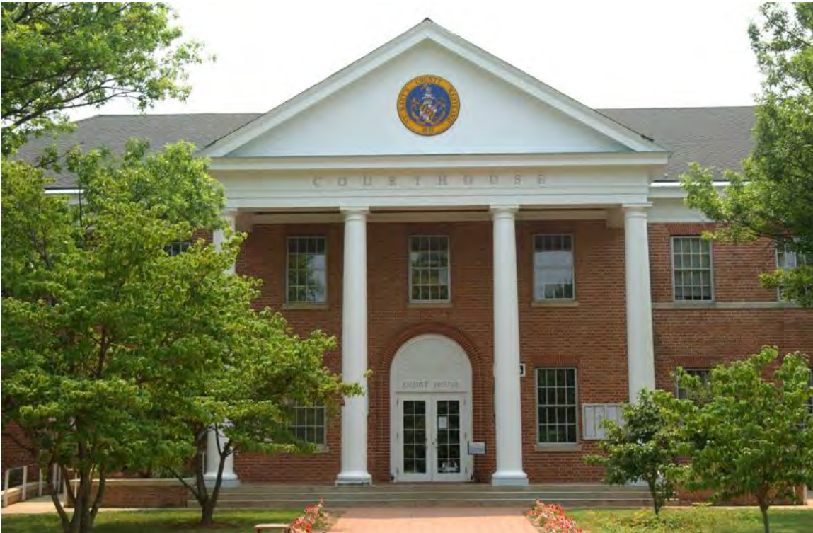
Circuit Court for St. Mary's County
